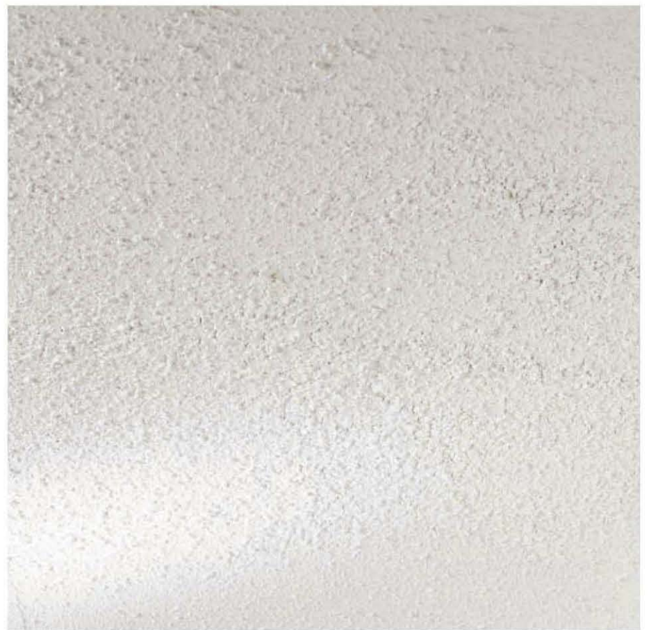
A popcorn ceiling is no treat if you are trying to sell a house (or just keep it clean, for that matter). The best thing about textured ceiling treatments is that they are easy to remove.
