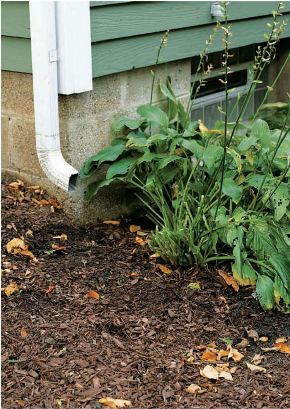
Gutter downspouts without extensions dump huge amounts of water right near the foundation, while an improper grade keeps surface water against the house. Downspout extensions and corrections to the grade solve many basement moisture problems.
