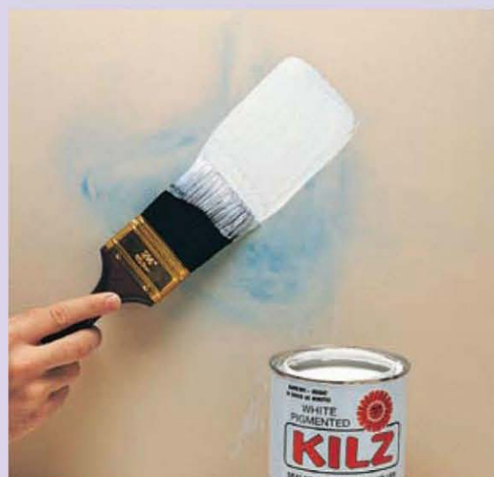
Seal all stain areas with white pigmented shellac. Pigmented shellac prevents stains from bleeding through the new paint.
