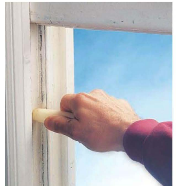
A white candle or block of paraffin wax is an all-purpose lubricant for wood windows. Never use liquid or greasy lubricants on wood windows.
