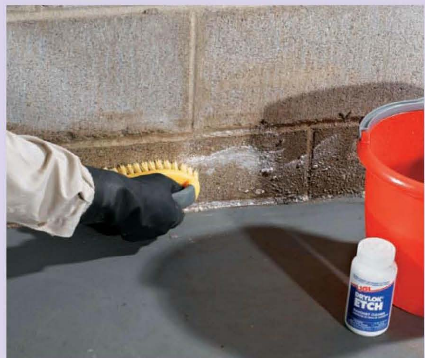
Remove efflorescence prior to coating a concrete or block basement wall. Make sure the cleaner is compatible with the wall coating; it's best if both come from the same manufacturer.
