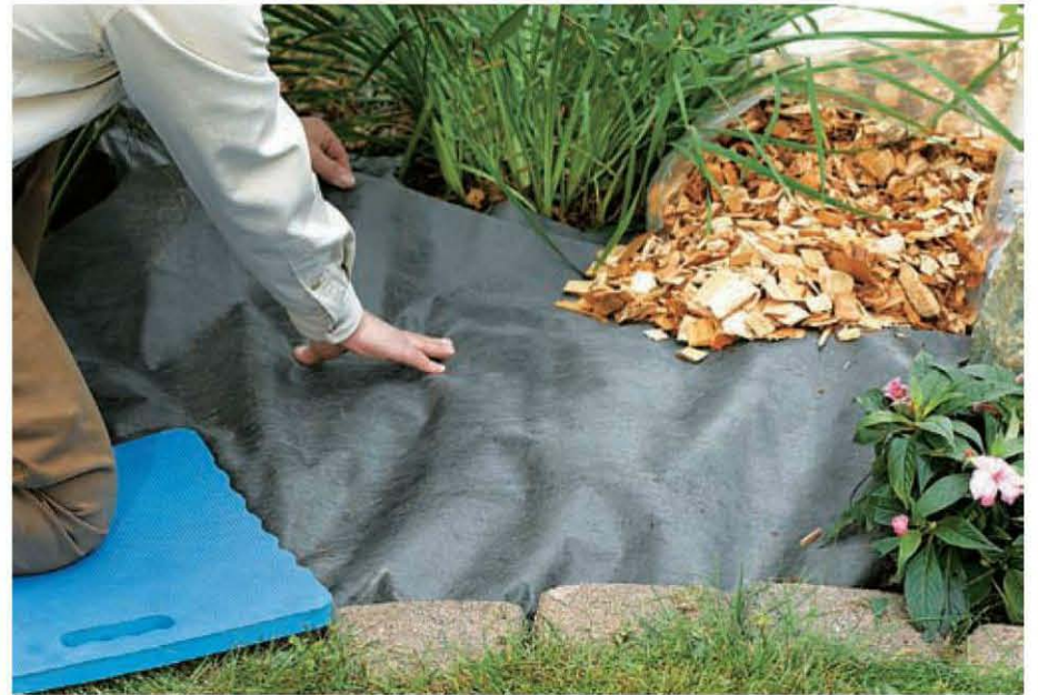
Landscape fabric and edging combine forces to control weeds, keep groundcover contained, and make mowing grass easier.
