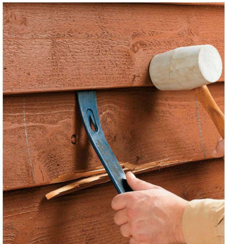
Some types of siding are nailed at the top and bottom edges, with each nail penetrating two pieces at once. Remove the nails by prying up the edge slightly, then hammering the board to pop the nail heads. This is especially useful for pulling the nails on the good pieces.
