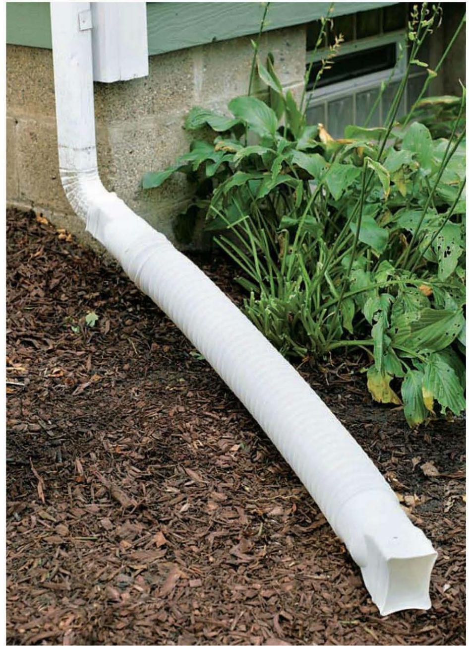
Gutter downspouts without extensions dump huge amounts of water right near the foundation, while an improper grade keeps surface water against the house. Downspout extensions and corrections to the grade solve many basement moisture problems.
