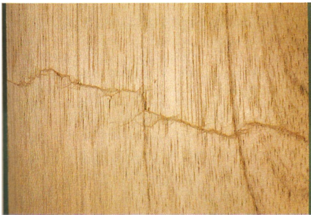
Figure 4.52 • Compression failures appear as wrinkles across the grain on the longitudinal surfaces of dressed lumber. Photo by Randy O'Rourke)
