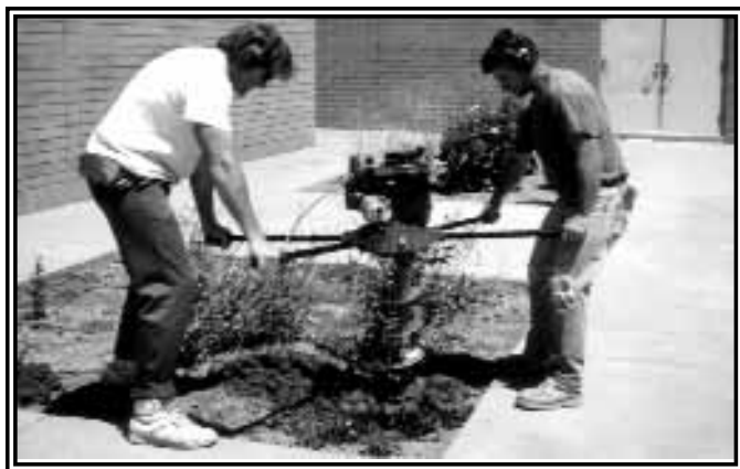
Drilling into the hard Arizona soil.
