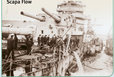
Salvage work at Scapa Flow
