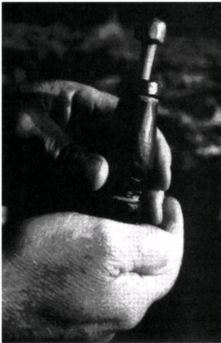
Fire piston cylinder made from buffalo horn with wooden piston. From Mel Dewese collection (Photo by Richard Jamison).
