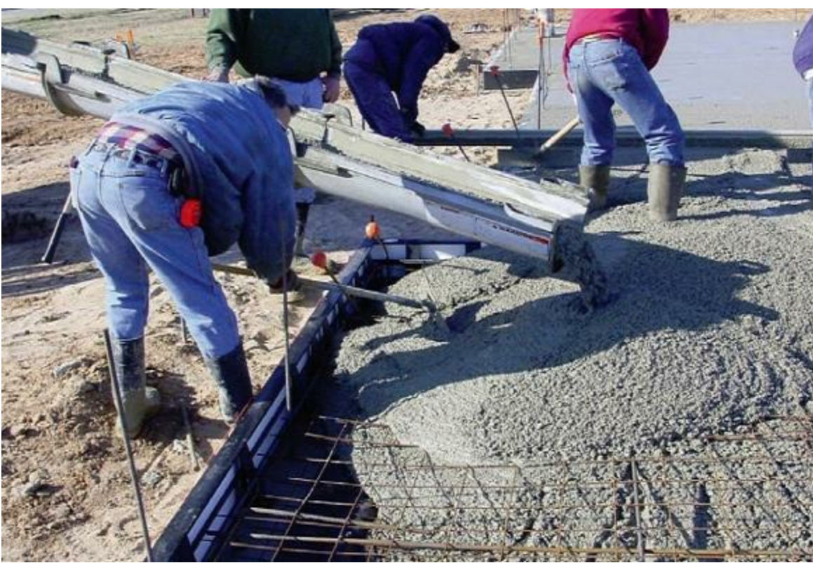
Figure 6.12 EnergyEdge-form concrete slab pouring.
