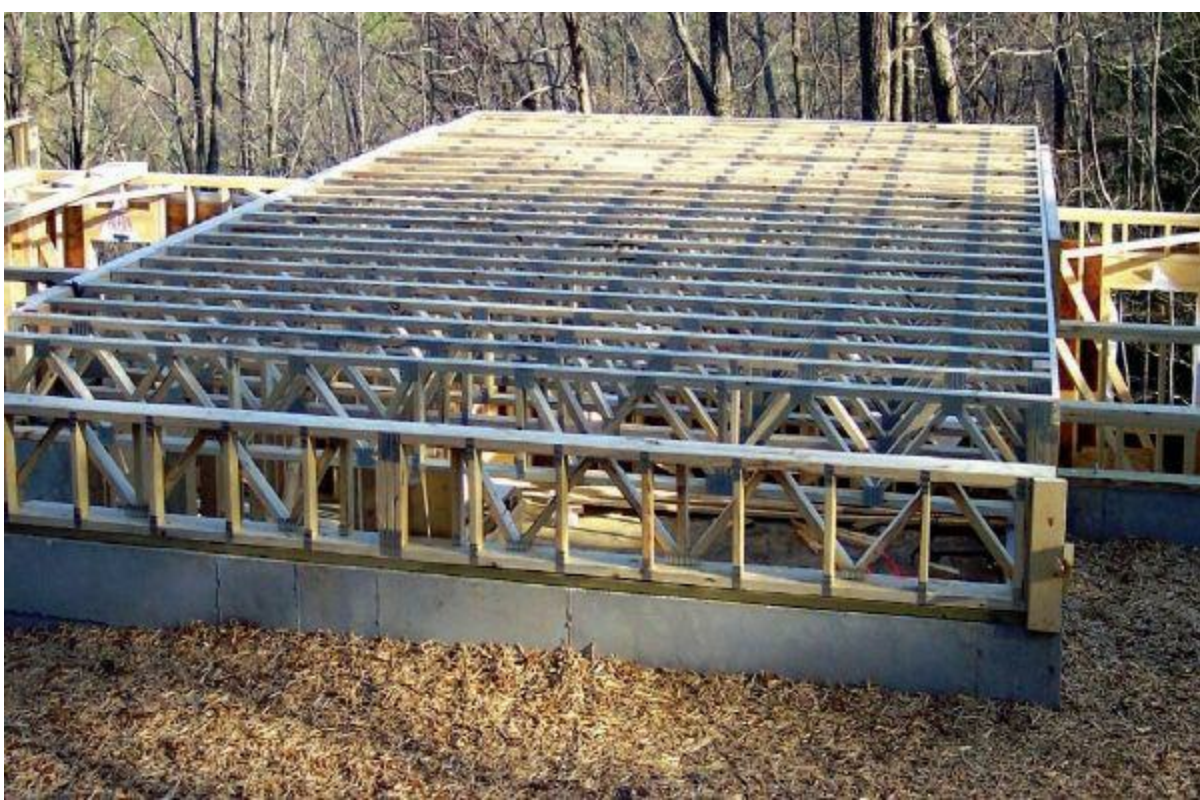
Figure 6.16 Floor trusses.
