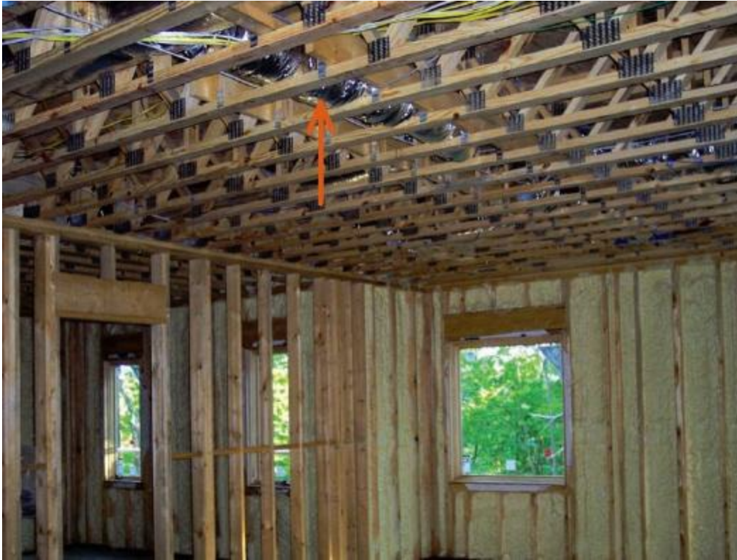
Figure 6.15 HVAC installed in floor trusses.
