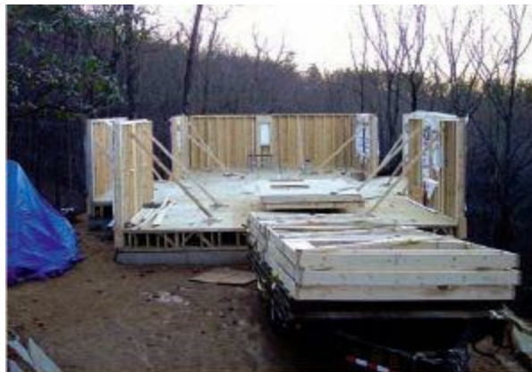
Figure 12.22 Most of the exterior walls are now erected.
