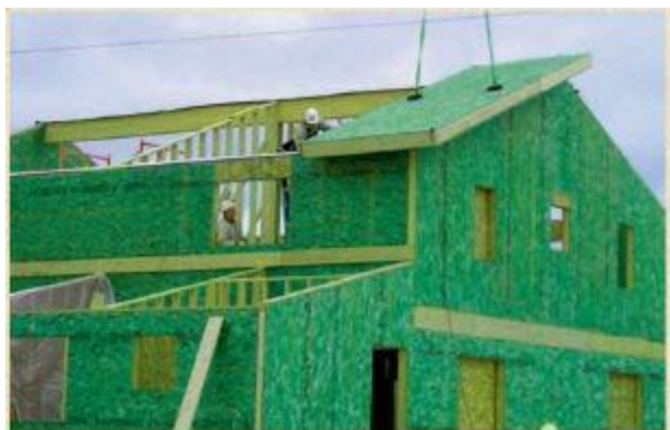
Figure 8.6 Larger SIP’s — roof with ridge beam.
