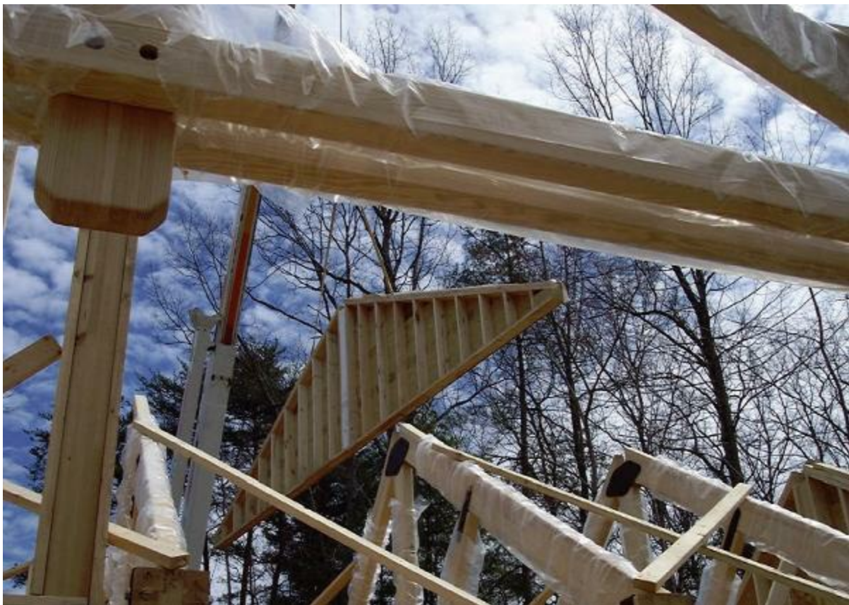
Figure 12.27 One of the matching Gable-end walls is being lifted in place.
