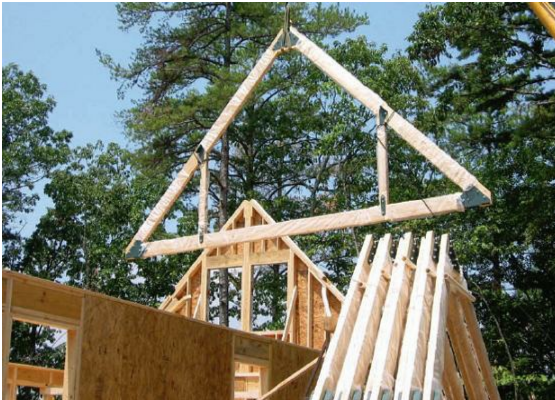
Figure 5.6 Loft trusses being lifted into place at mountain chalet.
