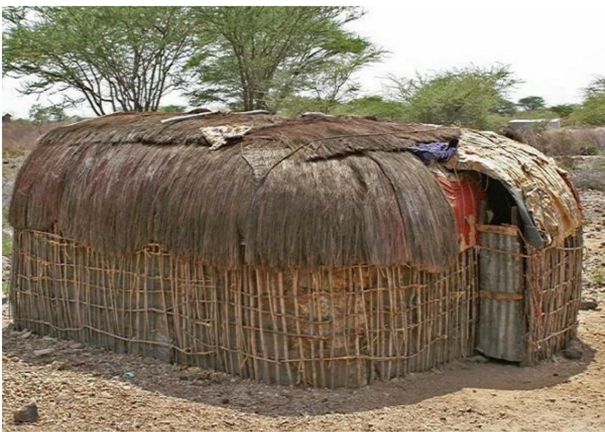
Figure 10.7 Another house in the same village north of Archer's Post, Kenya. The women design and build their homes. Part of this roof is made from a reed-like material gathered from the foot of a "nearby" (about a 20-mile/30-35km walk) mountain. The builder said this roof is very good and will last a long time. (PHOTO BY JIM STACK)
