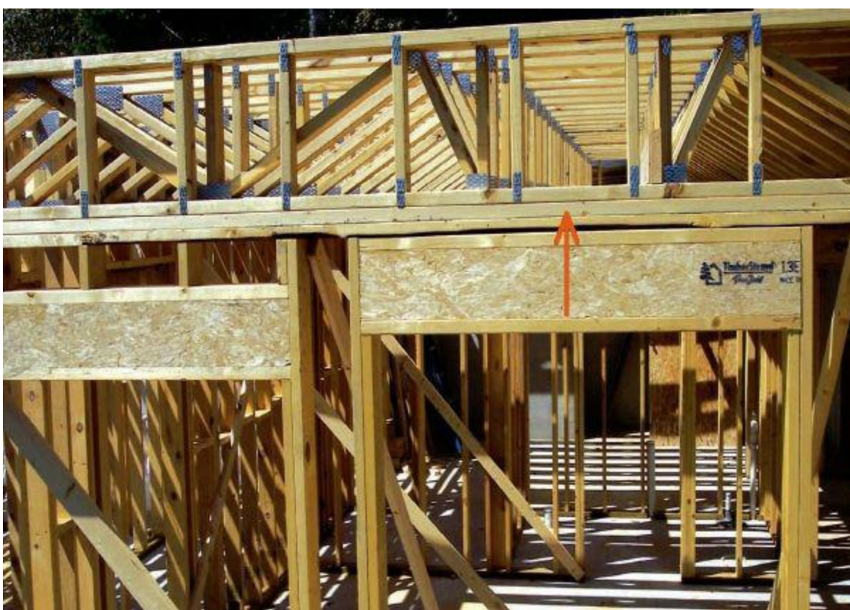
Figure 6.14 HVAC chase in floor trusses.
