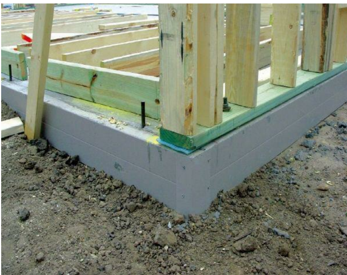
Figure 6.10 EnergyEdge-form example on slab edge.
