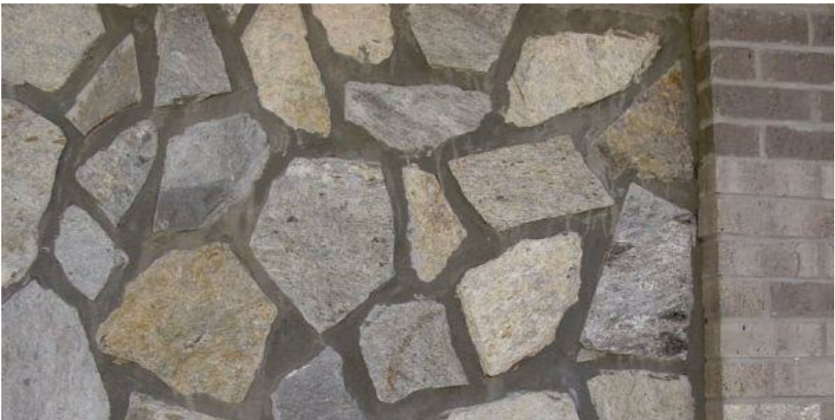
Figure 10.2 Brick and stone combination.
