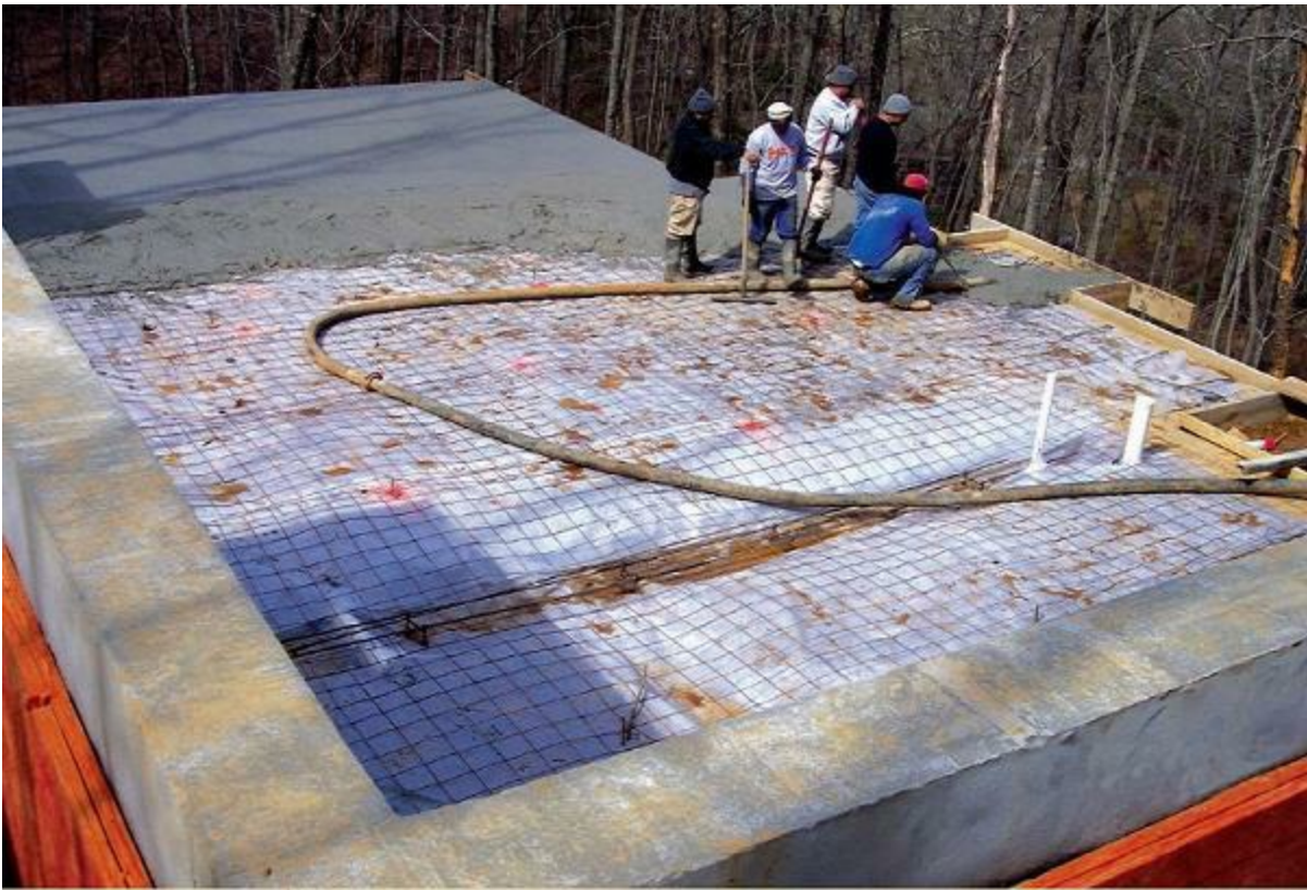
Figure 12.13 The basement slab.
