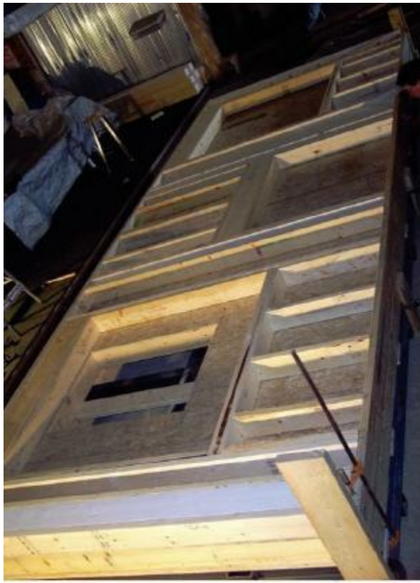
Figure 12.15 Pre-built walls sections in shop.
