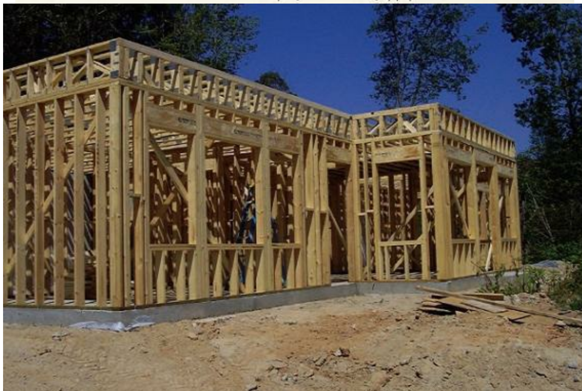
Figure 6.9 Exposed basement slab edge
