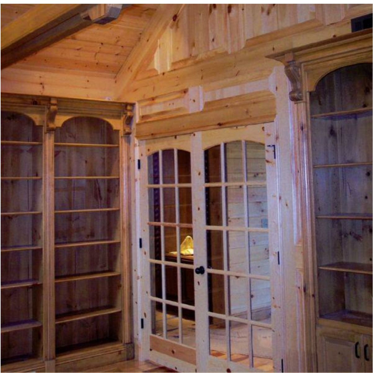
Figure 10.1 Interior French doors.
