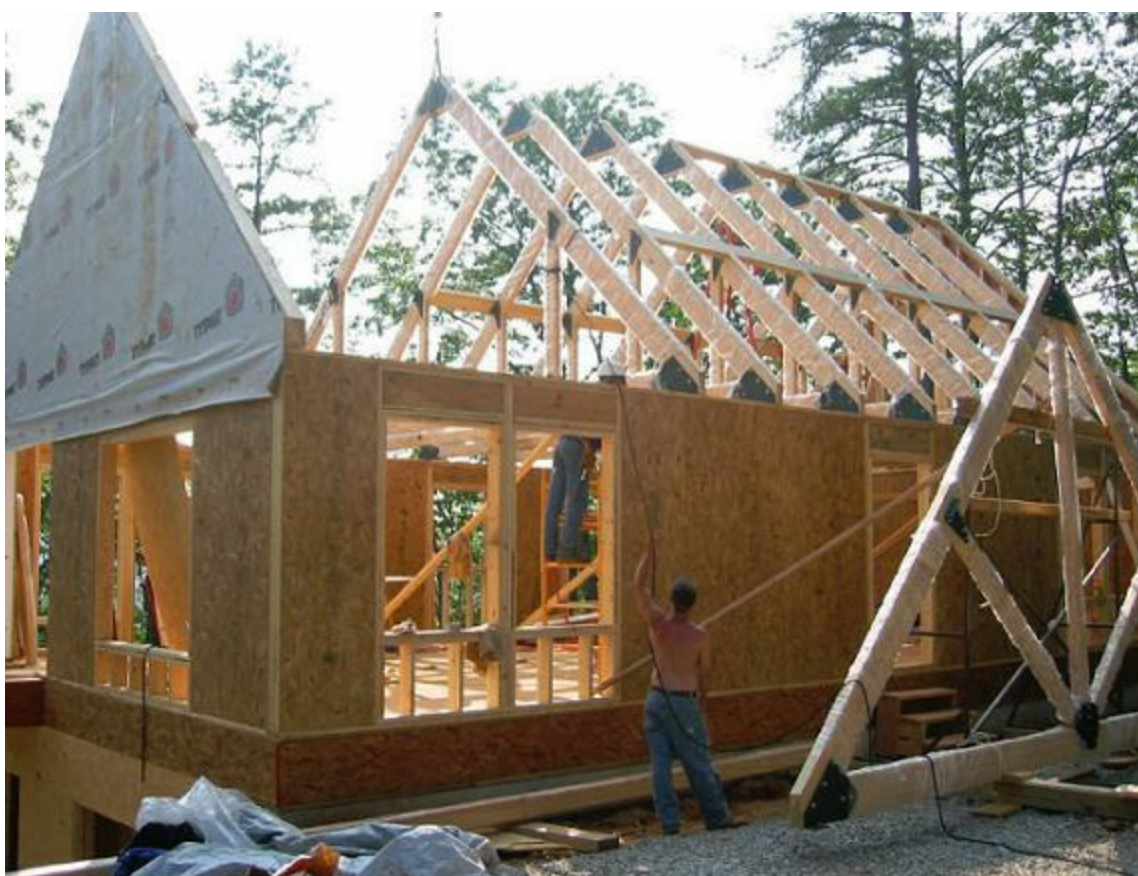
Figure 8.2 SIP walls and timber-truss style.
