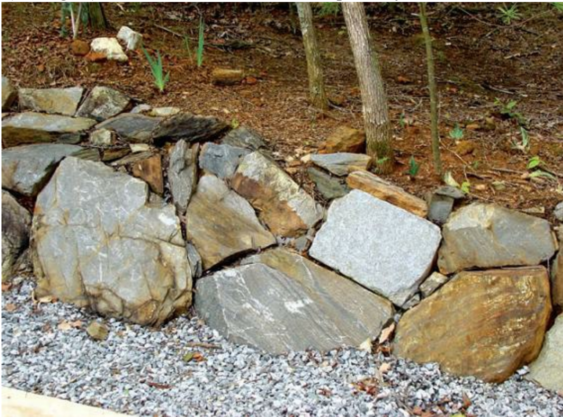
Figure 11.4 Local, natural-rock retaining wall.
