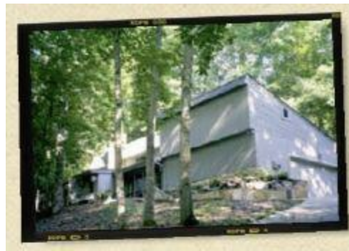
Figure 6.1 Suburban Atlanta passive-solar home.
