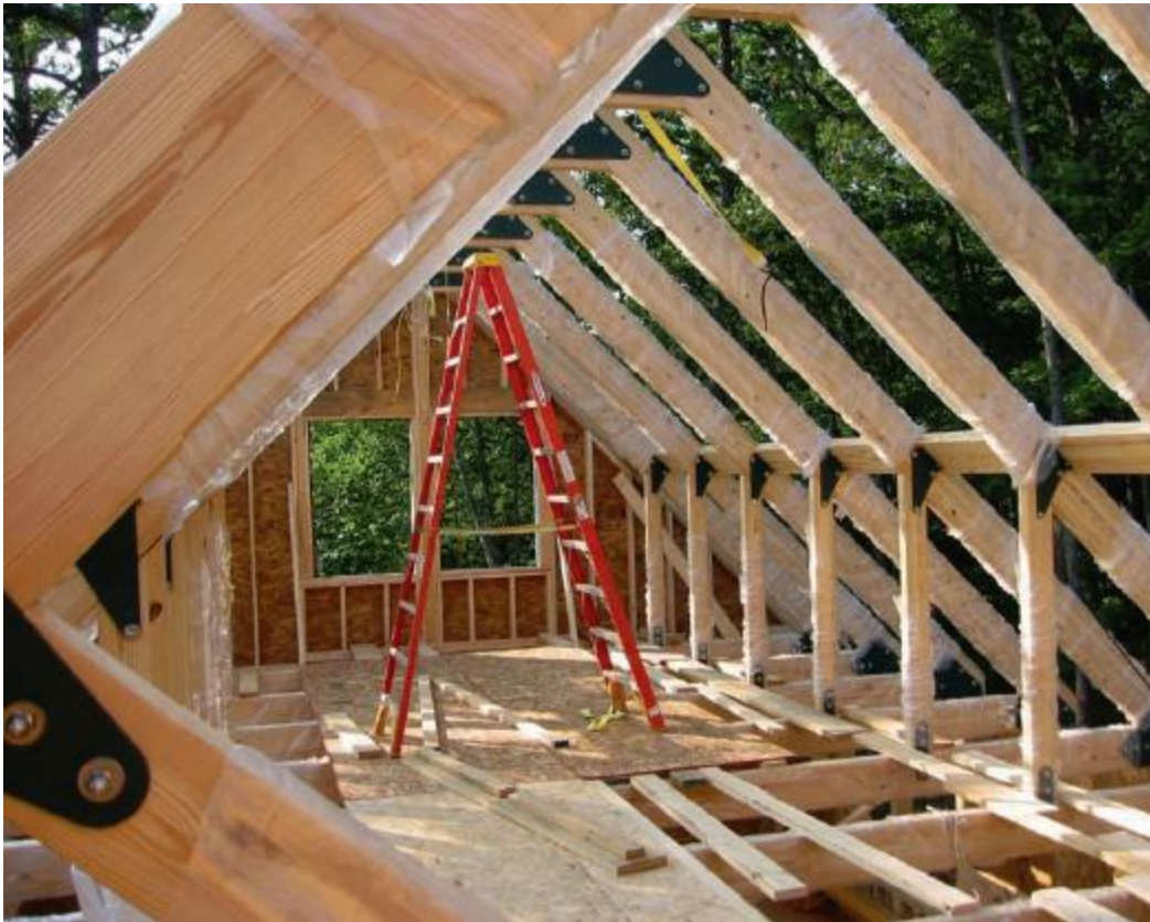
Figure 5.7 Loft trusses prior to the 2×4 T&G paneling.
