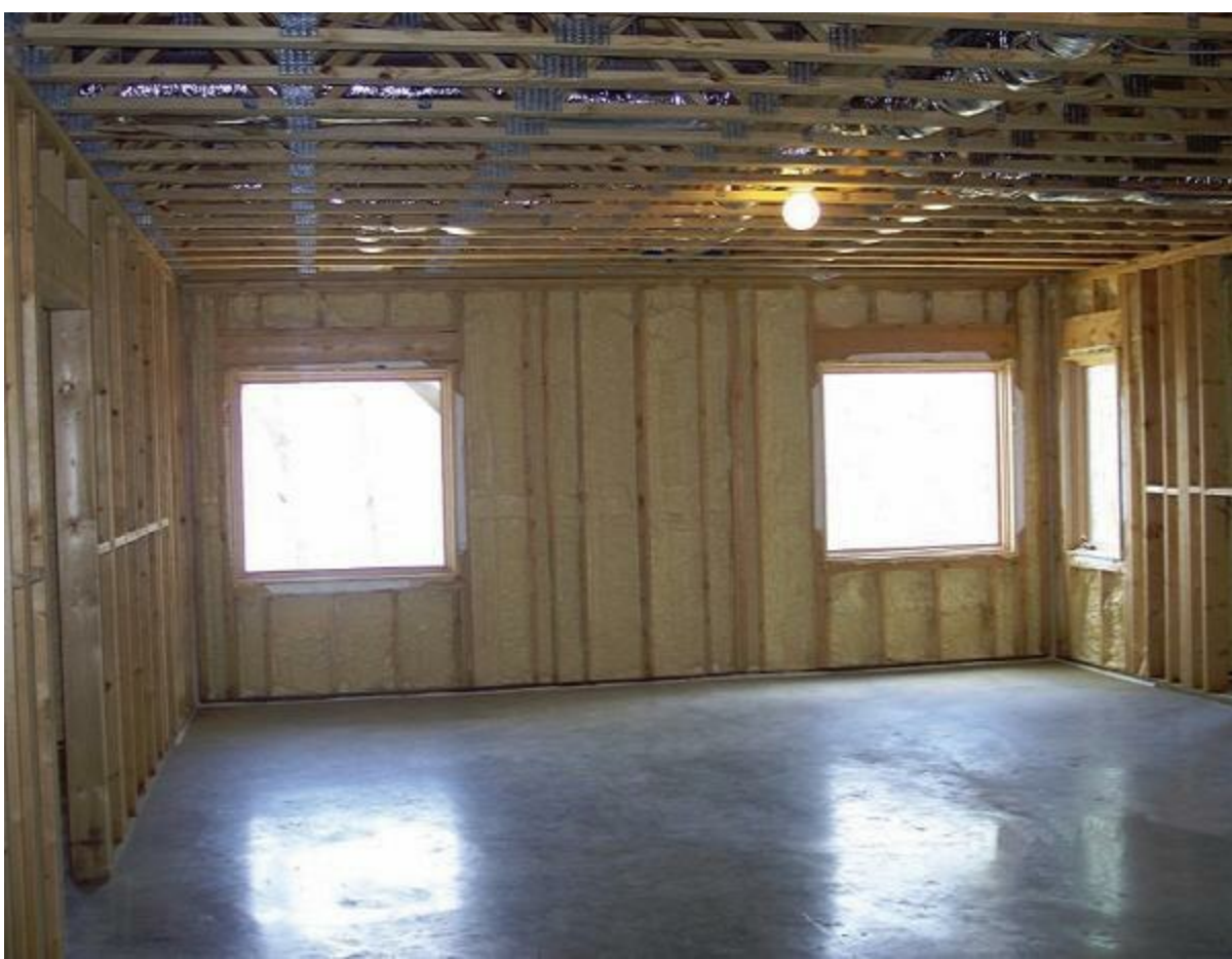
Figure 12.11 Energystar house basement den wall.
