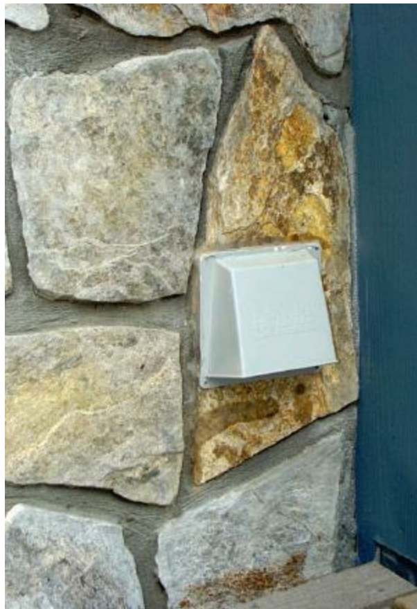
Figure 6.20 Direct-combustion air intake for fireplace.
