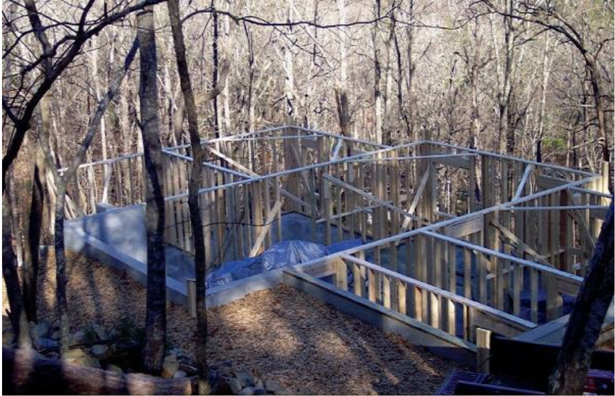
Figure 12.17 Basement framing is finished.
