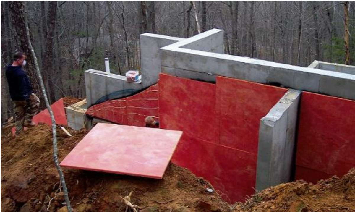
Figure 12.14 Energystar house warm-and-dry installation.
