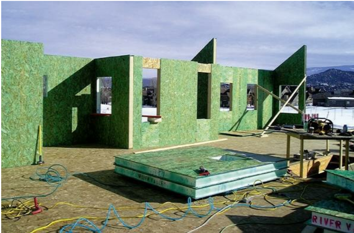
Figure 8.5 Larger SIP’s for walls.
