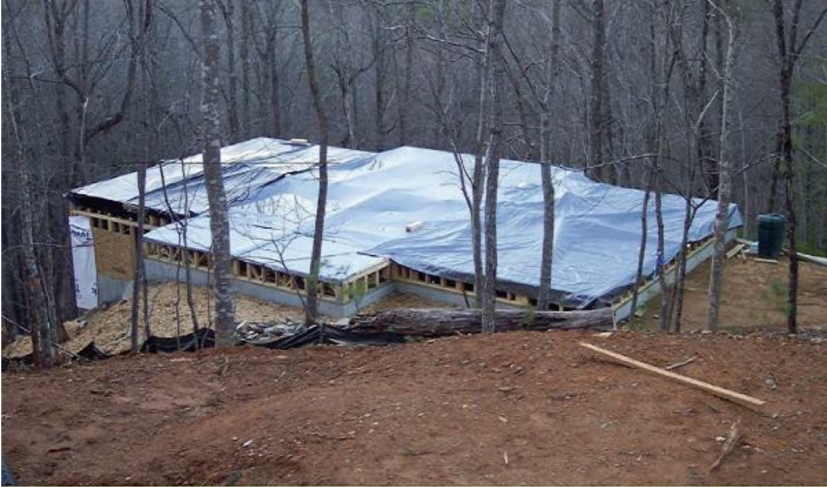
Figure 12.19 Floor decking (covered).
