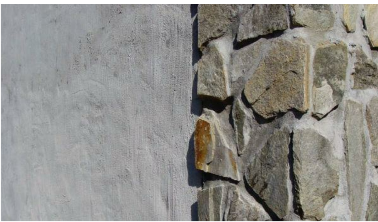
Figure 10.3 Garage stone corner and stucco wall.
