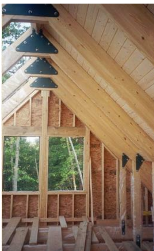
Figure 5.8 Loft decking partially installed.
