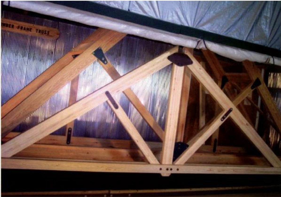
Figure 7.7 Timber truss in the shop.
