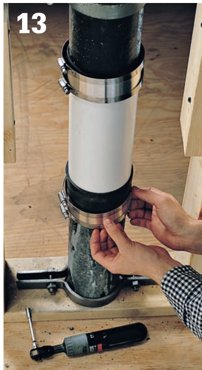
13 Slide stainless-steel bands and clamps over the neoprene sleeves.
