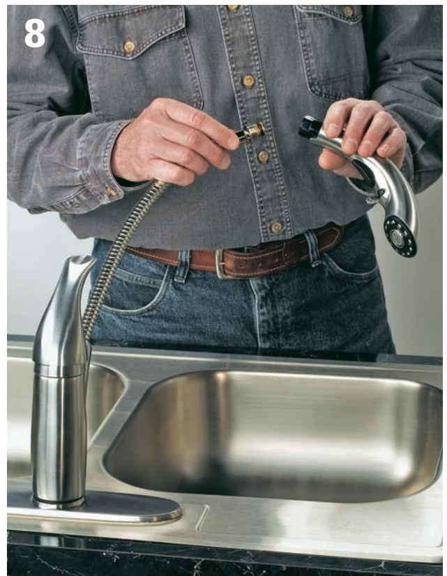
8 Attach the spray head to the end of the pullout hose and turn the fitting to secure the connection. Turn on water supply and test. Tip: Remove the aerator in the tip of the spray head and run hot and cold water to flush out any debris.
