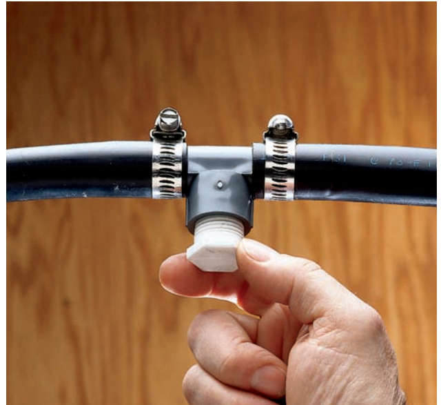
Connect lengths of PE pipe with a barbed PVC fitting. Secure the connection with stainless steel hose clamps.
