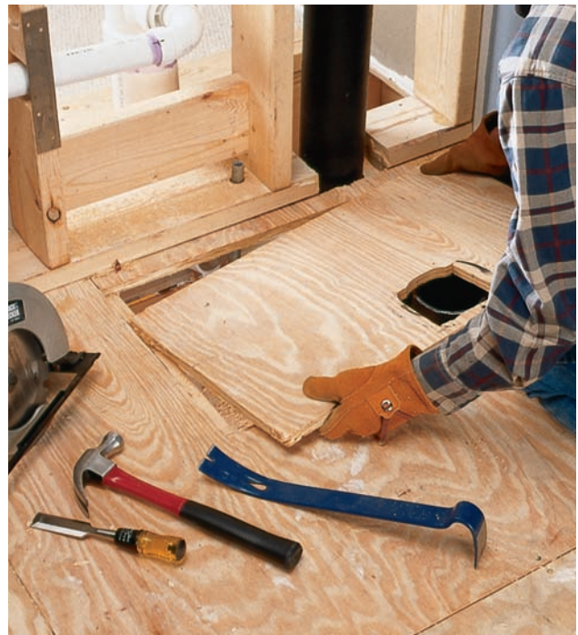
Replacing a toilet drain usually requires that you remove flooring and wall surface to gain access to the pipes.
