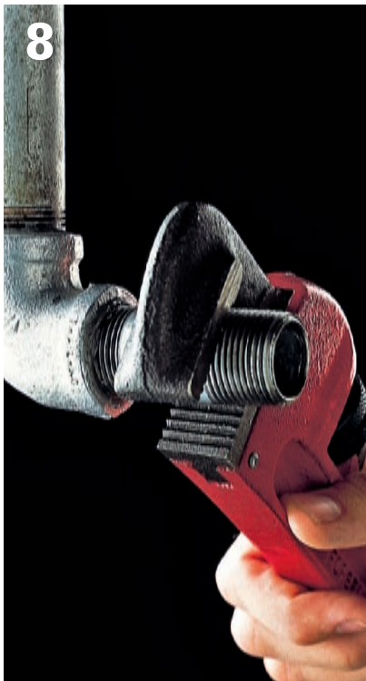
8 Screw the first nipple into the fitting, and tighten with a pipe wrench.
