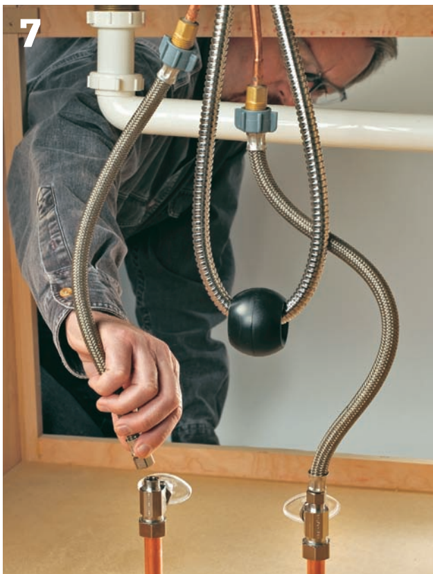
7 Connect the supply tubes to the supply risers at the stop valves. Make sure to get the hot lines and cold lines attached correctly.
