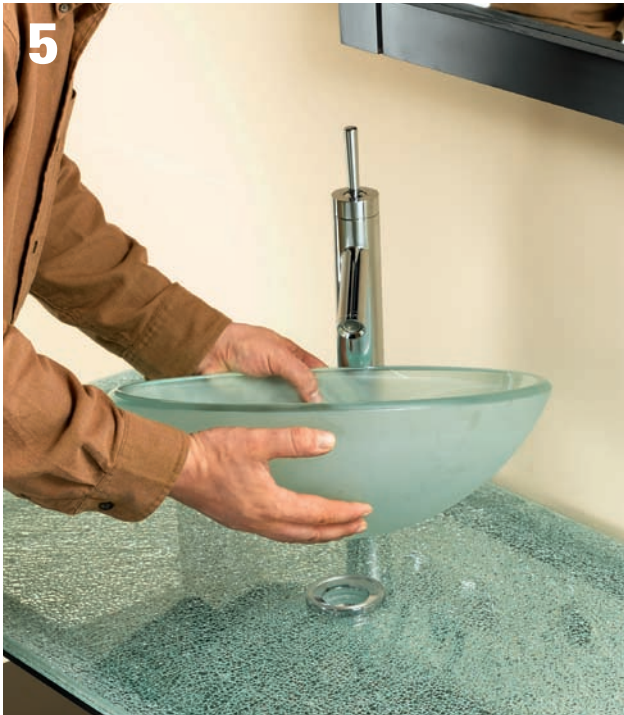
5 Place the vessel bowl on top of the O-rings. In this installation, the vessel is not bonded to the countertop.
