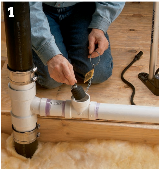
Insert a test balloon into the test T-fittings at the top and bottom of the new DWV line, blocking the pipes entirely. Note: Ordinary T-fittings installed near the bottom of the drain line and near the top of the vent line are generally used for test fittings.
