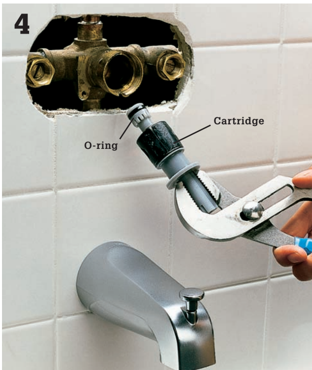
4 Remove the cartridge assembly by grasping the end of the valve with channel-type pliers and pulling gently.
