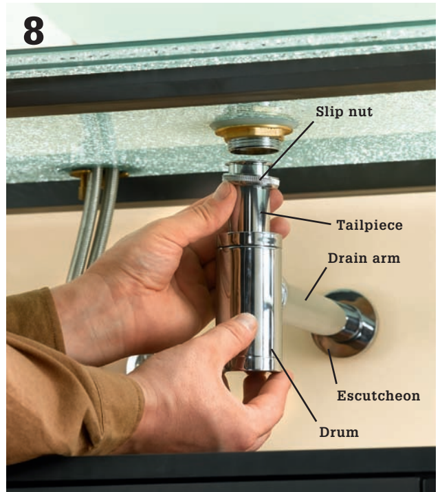
8 Install the drum trap. Loosen the rings on the top and outlet of the drum trap. Slide the drum trap top hole over the tailpiece. Slide the drain arm into the side outlet, with the flat side of the rubber gasket facing away from the trap. Insert the drain arm into the wall outlet. Hand tighten the rings.
