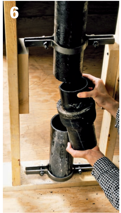
6 Repeat cutting at the other chalkline. Remove cut section of pipe.
