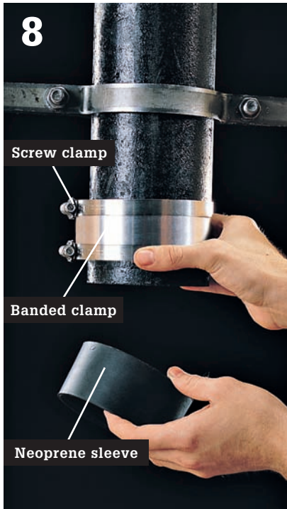
8 Slip a banded coupling and a neoprene sleeve onto each end of the cast-iron pipe.
