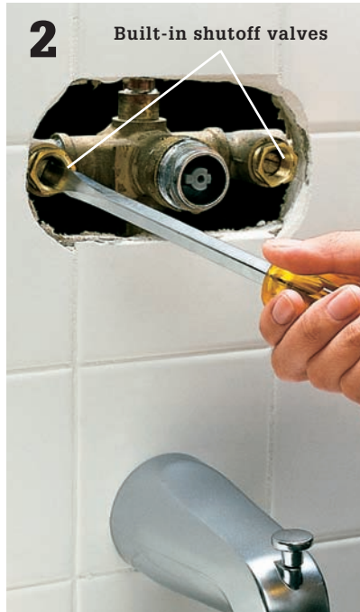
2 Turn off water supply at the built-in shutoff valves or the main shutoff valve.
