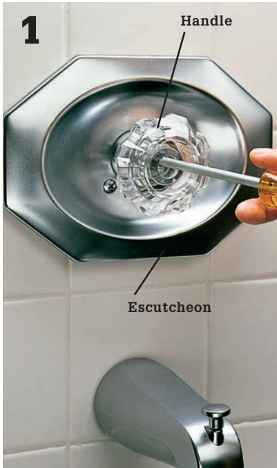
1 Use a screwdriver to remove the handle and escutcheon.
