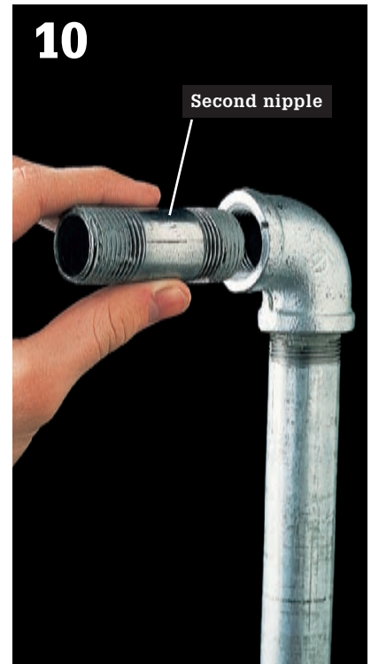
10 Screw the second nipple onto the other fitting. Tighten with a pipe wrench.
