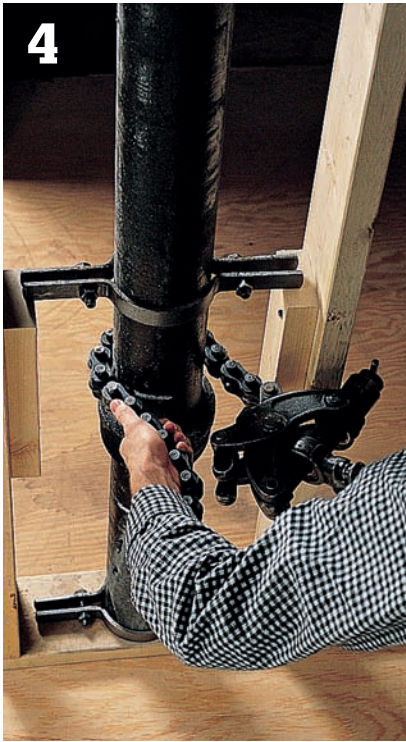
4 Wrap the chain of the snap cutter around the pipe, so that the cutting wheels are against the chalkline.
