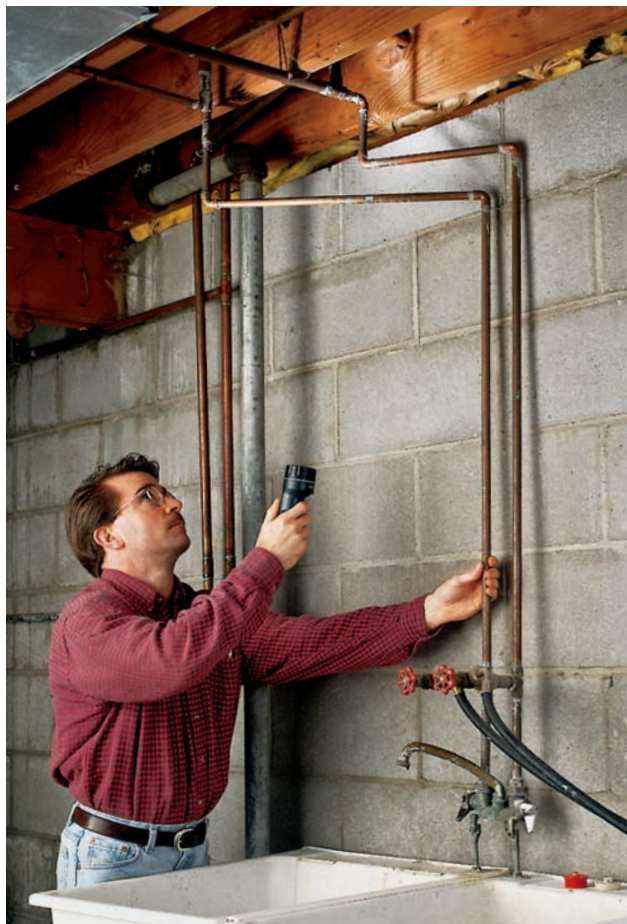
Snoop around your basement for clues about the locations of supply, drain, vent, and gas pipes in your walls.
