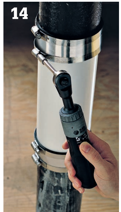
14 Tighten the screw clamps with a ratchet wrench or screwdriver.
