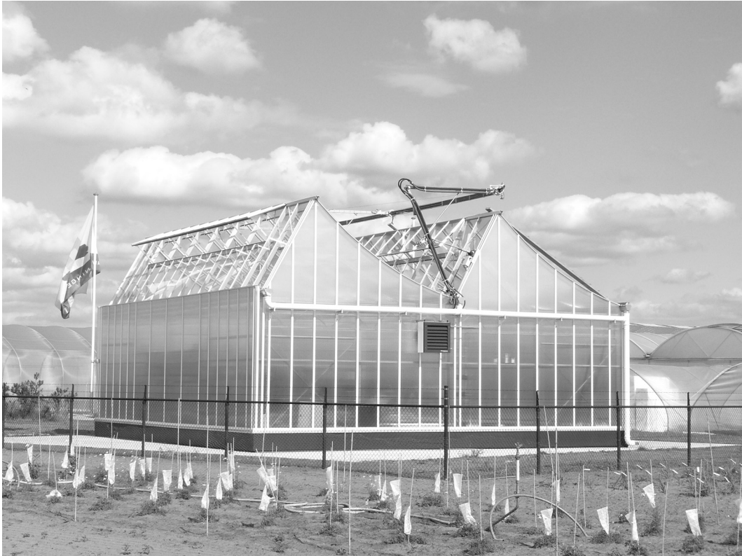
FIGURE 9.2 Electricity-producing greenhouse. (Courtesy of the Business Unit Glass, Plant Research International.)
