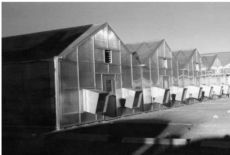
Figure 12.6 Placement of exhaust fans at the end of greenhouse (normal arrangement for pulling air into the greenhouse from openings in the opposite end of the greenhouse). Normally, exhaust fan placement is at the base of the greenhouse. For cross-flow ventilation, fans may be placed higher on the side walls, as in Figure 12.16.
