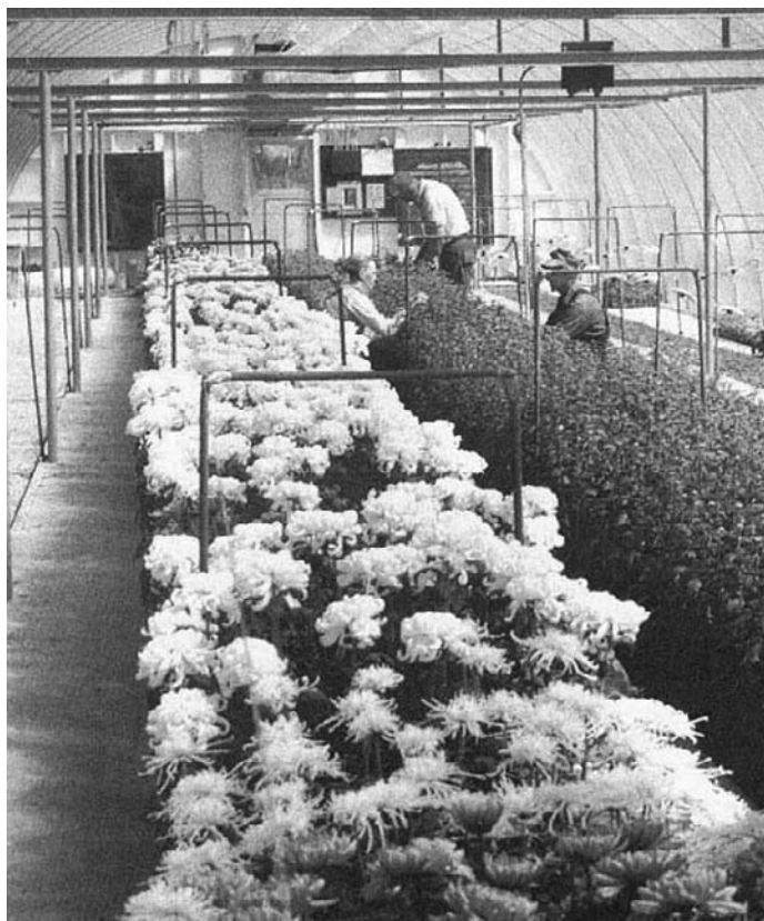
Figure 11.1 Gravel bed flood-and-drain hydroponic growing system designed for tomato greenhouse production that was successively switched to chrysanthemum flower production using the same growing procedures as for tomato. On the far left (just beyond the walkway) is a gravel bed ready to be planted.
