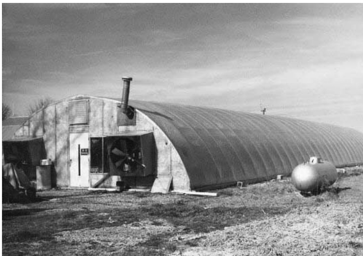
Figure 12.4 Quonset-style greenhouse (common design for most single-bay greenhouses primarily for use by an owner/grower operator).
