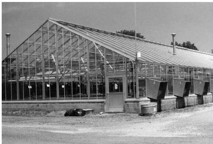
Figure 12.11 Ventilation vents at the roof ridge line open to allow hot air to be exhausted from the greenhouse gable.
