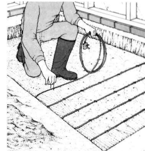
2 Lay soil heating cables on the soil surface. Space the cable in a series of loops 4-6 in apart. Do not let the loops touch. Peg the cable down with staples.
