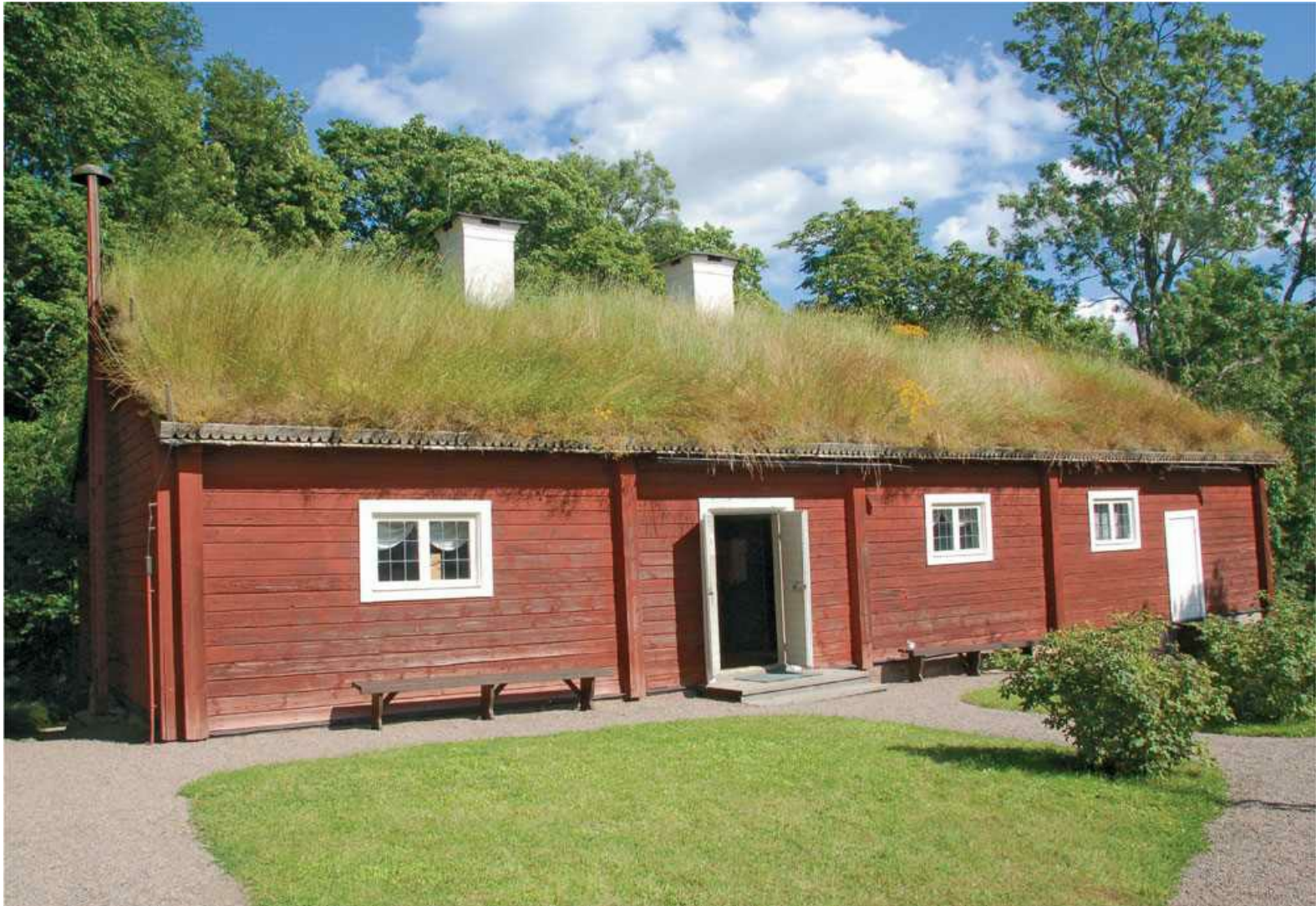
A green roof can be made up of low-growing groundcovers or even grass.
