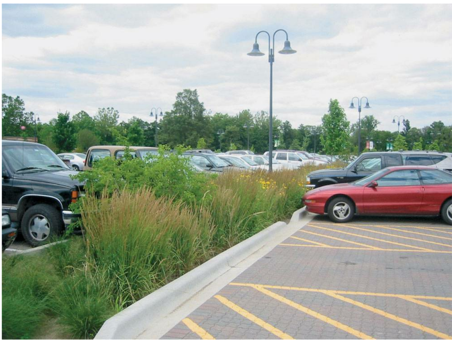
Rain gardens can be used as valuable green spaces in parking lots.
