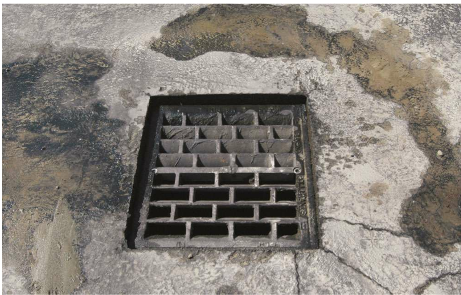
Catch basin grates should be placed in low areas where water collects.
