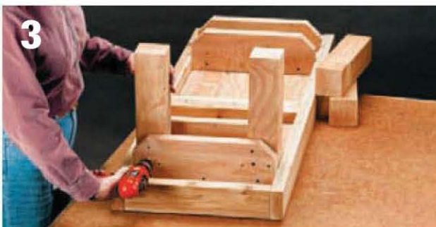
3 Position each leg between a set of braces and against the sides of the bench frame. Drill pilot holes through each brace and attach the leg to the braces.
