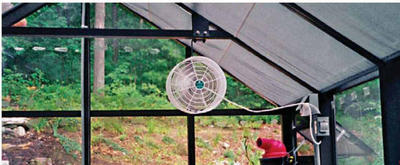
Roof shades , along with vents, help prevent a greenhouse from overheating in direct sunlight. Here, a combination of circulating fans and cloth shades mounted on the interior of the south-facing glass helps protect plants.
