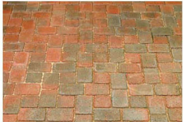
Concrete pavers set in sand offer a longlasting, stable floorcovering that breathes and allows for good drainage.
