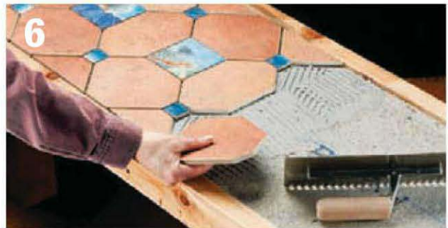
Set the tiles into the thinset mortar using a slight twisting motion as you press down.
