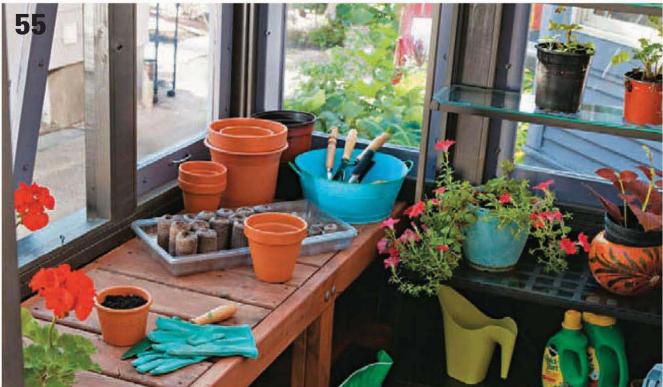
Finish the interior. You may add interior wallcoverings if you wish, but the exposed stud bays are good spots for adding shelving. For instructions on building this built-in potting bench, see pages 134 to 137.
