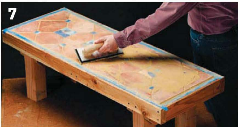
Mix a batch of grout and use a grout float to force it into the joints between tiles. Buff off the excess once the grout sets up.
