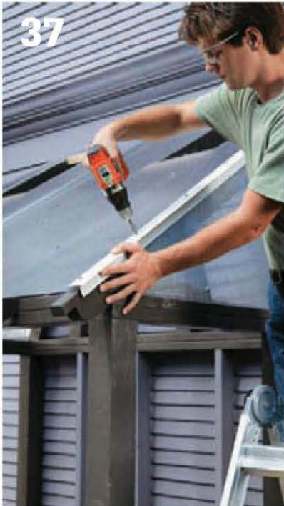
37 Install flashing over the hip roof seams. Here, common drip cap flashing is being fastened with rubber-gasket screws driven into the roof rafters.
