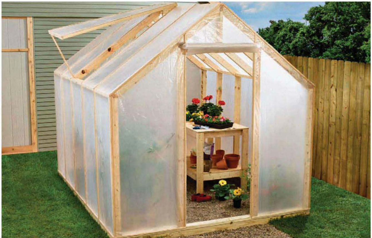
An A-frame greenhouse is easy to design and build yourself with just some wood and sheet plastic. See page 72.
