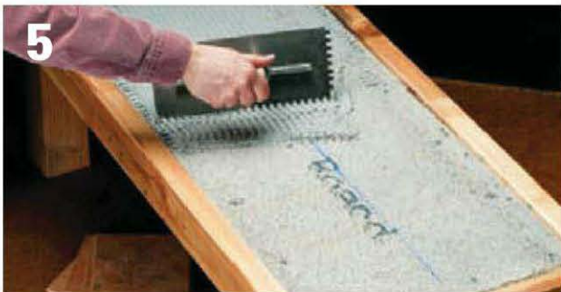
Apply a setting bed of thinset mortar onto the cementboard using a notched trowel.
