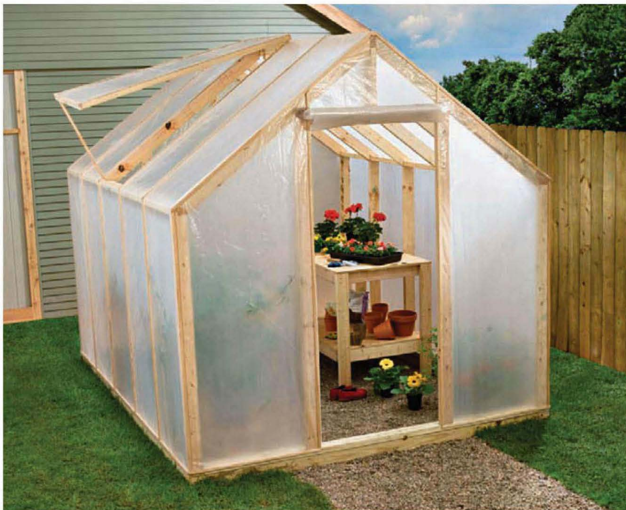
A wood-frame greenhouse with sheet-plastic cover is an inexpensive, semipermanent gardening structure that can be used as a potting area as well as a protective greenhouse.
