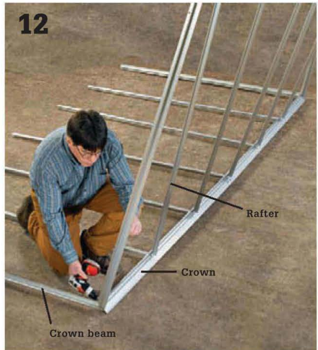
12 Assemble the roof frame on a flat area near the wall assembly. First assemble the crown-beam pieces; then attach the rafters to the crown, one by one. The end rafters, called the crown beams, have a different configuration, so make sure not to confuse them.
