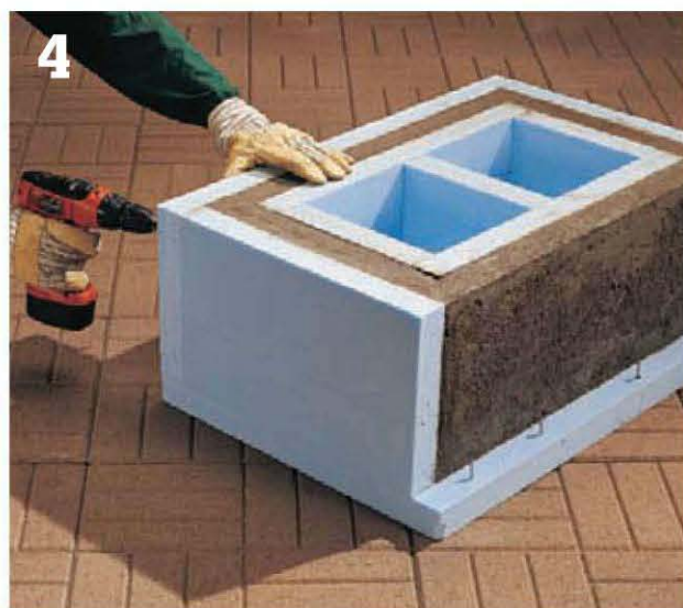
After the planter has dried for 48 hours, remove the screws and carefully disassemble the forms.
