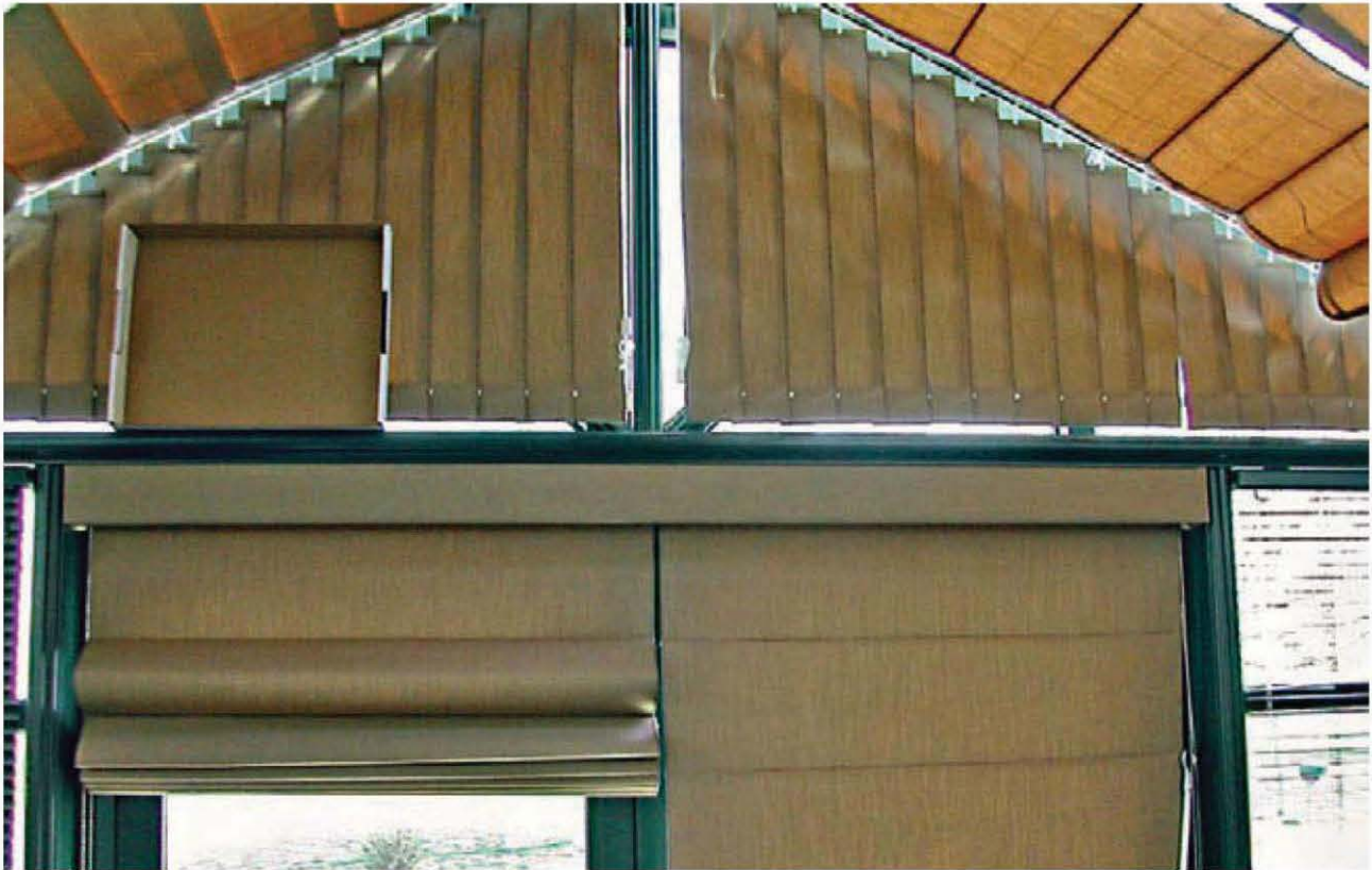
Louvered and roll-up shades help to block the sun in this greenhouse.
