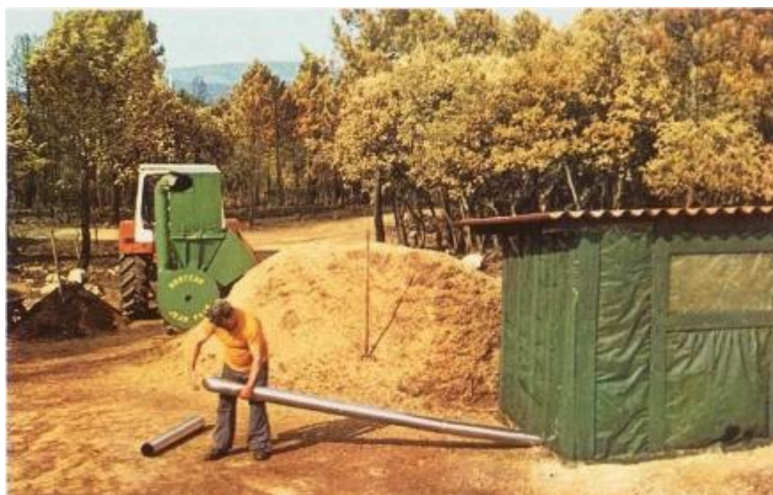
An opening was made at the bottom of the shed, at ground level, and the sections of piping fitted...
