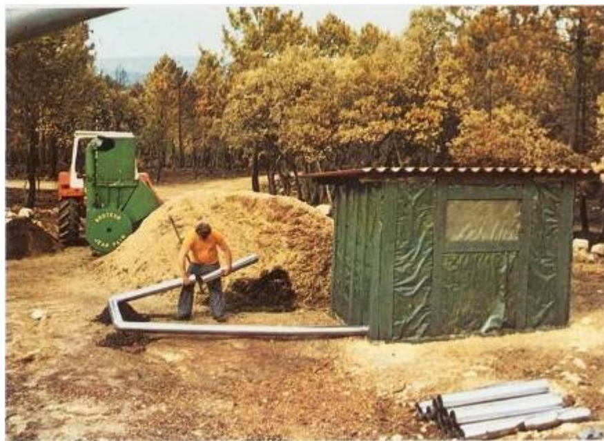
... Into one other and fixed together by elbow-shaped bends...
