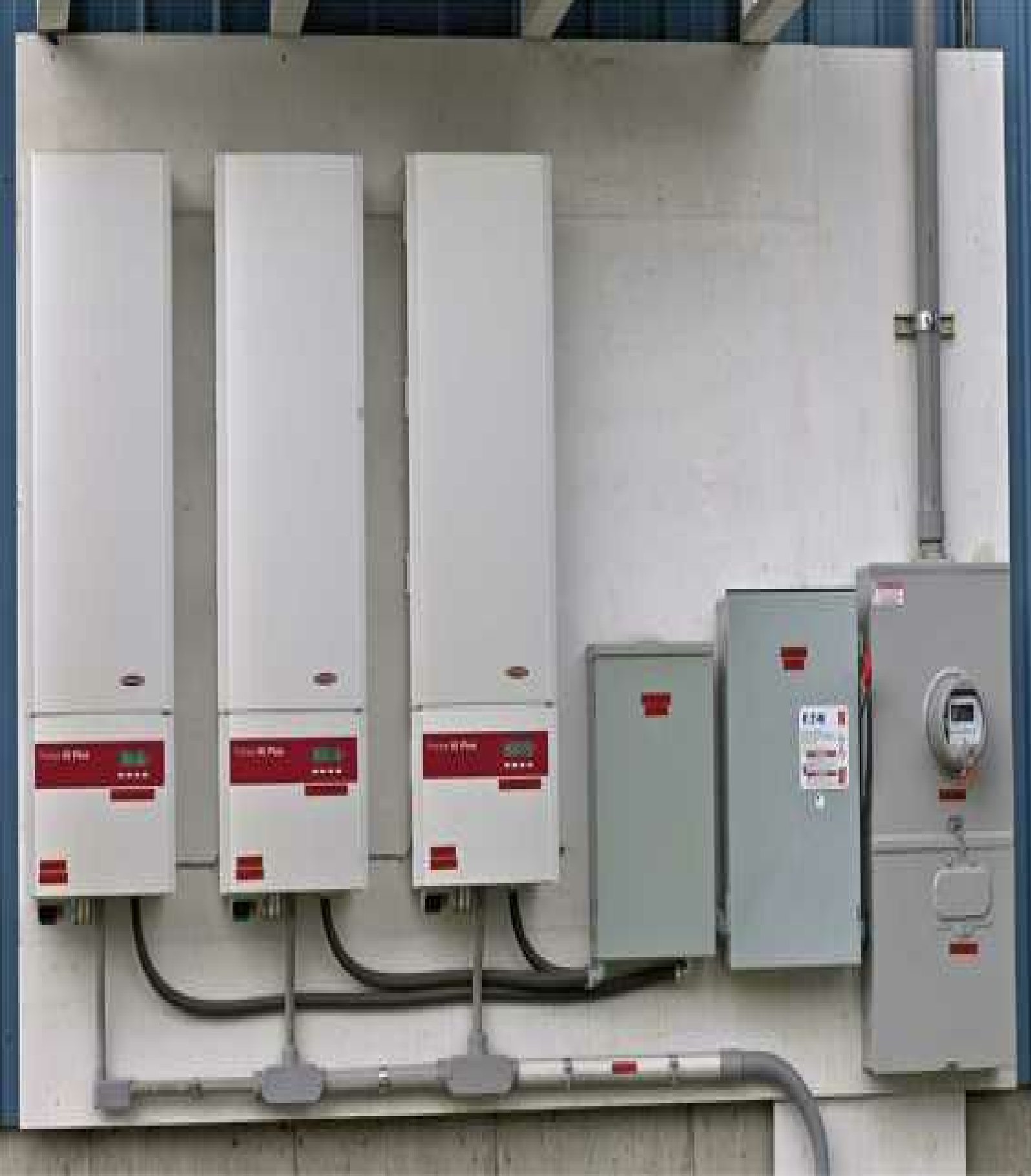
FIGURE G-24 A utility-interactive synchronous inverter. (Courtesy of Kaco.)
