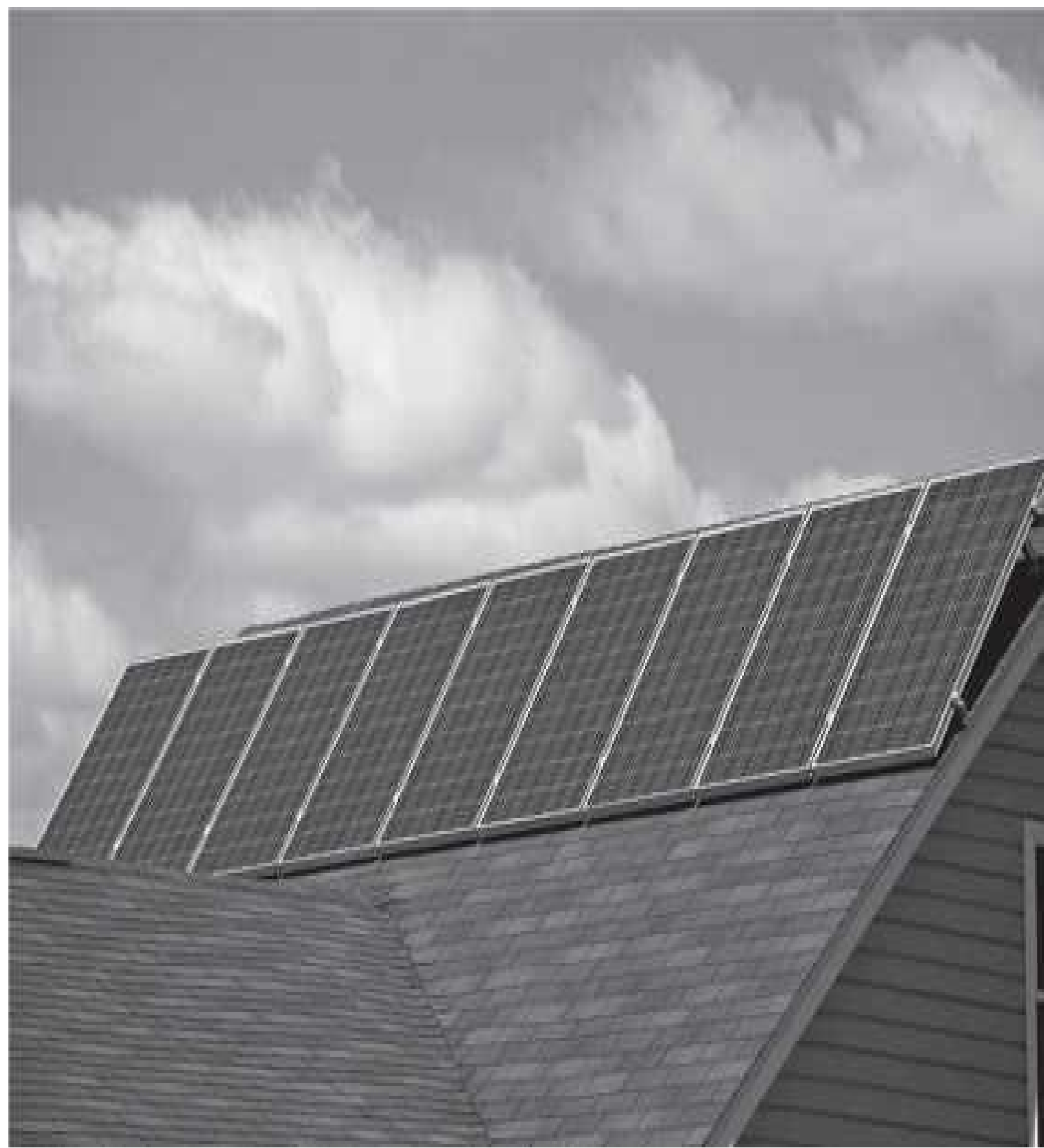
FIGURE 14-3 A roof-mounted solar array is unobtrusive.
