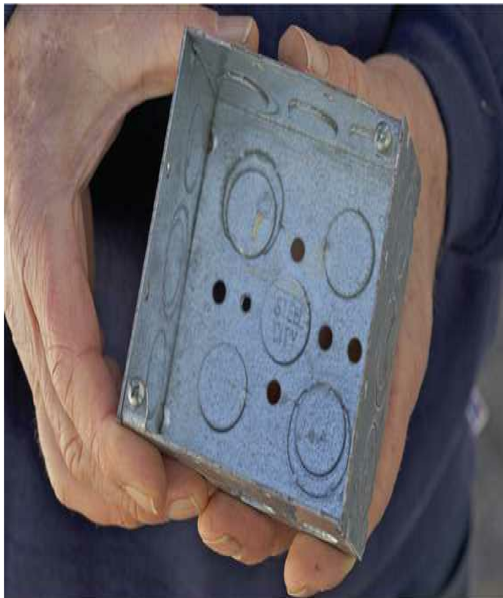
FIGURE 5-8 Large enclosures make for less box fill so that the installation is compliant and there is no chance of conductor damage.
