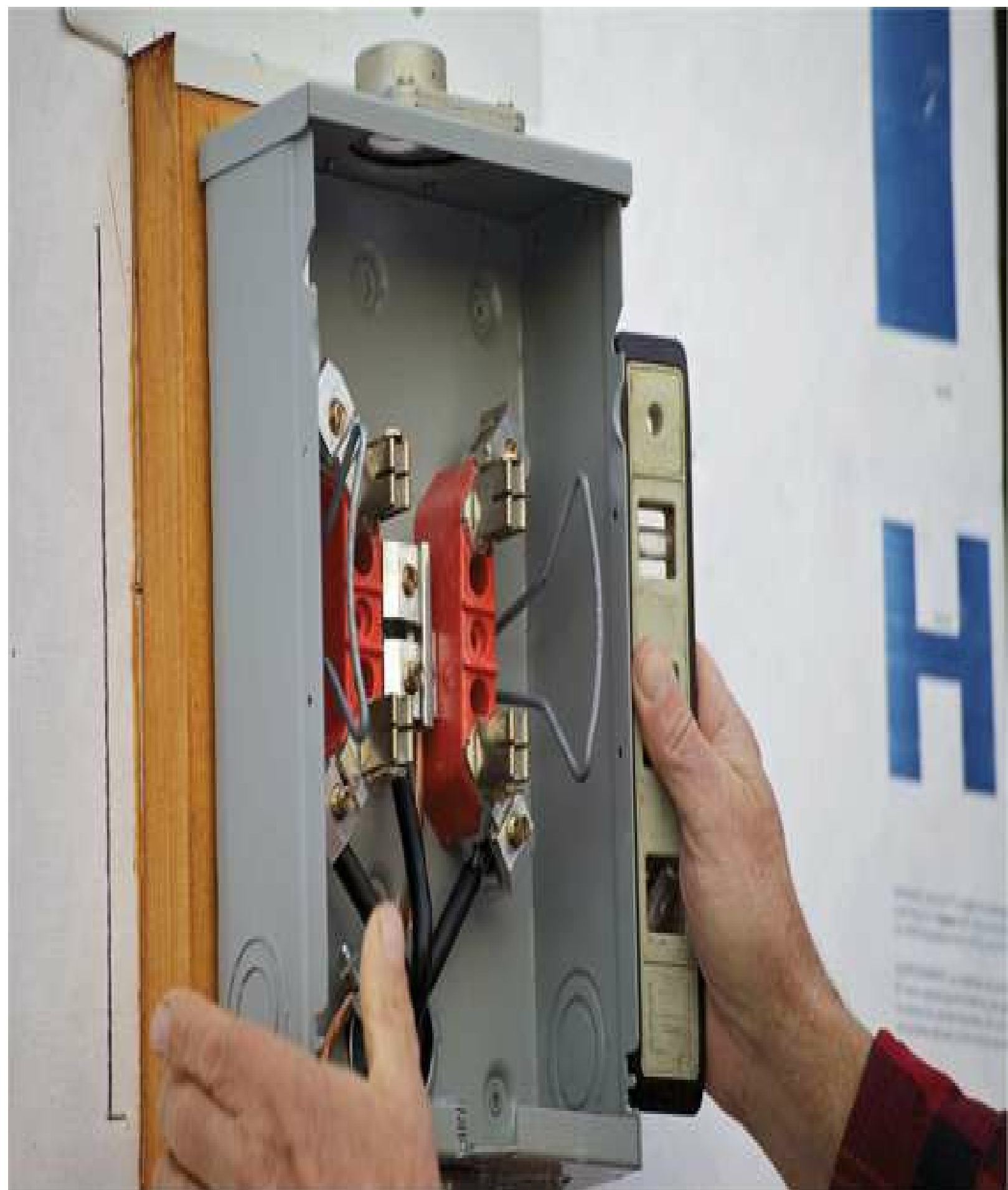
FIGURE 4-2 The utility will have definite ideas regarding meter location. It is central to the design of the service.
