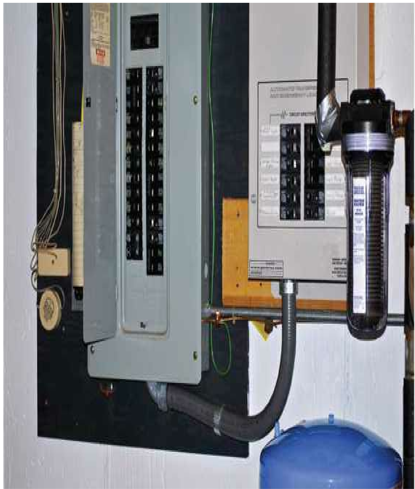
FIGURE 5-4 Note the clear violation of working-space requirements.
