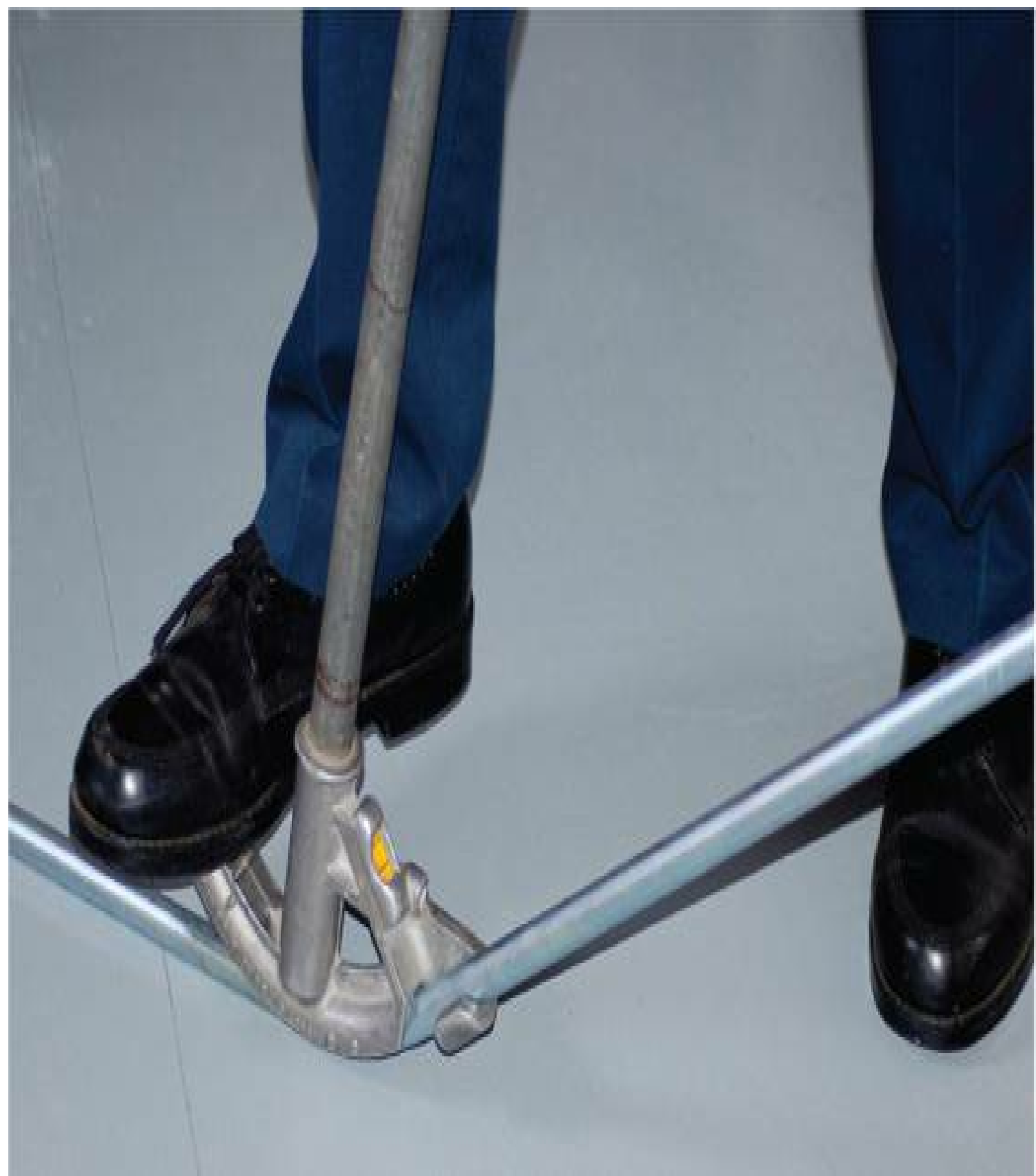
FIGURE 7-11 Bending EMT.
