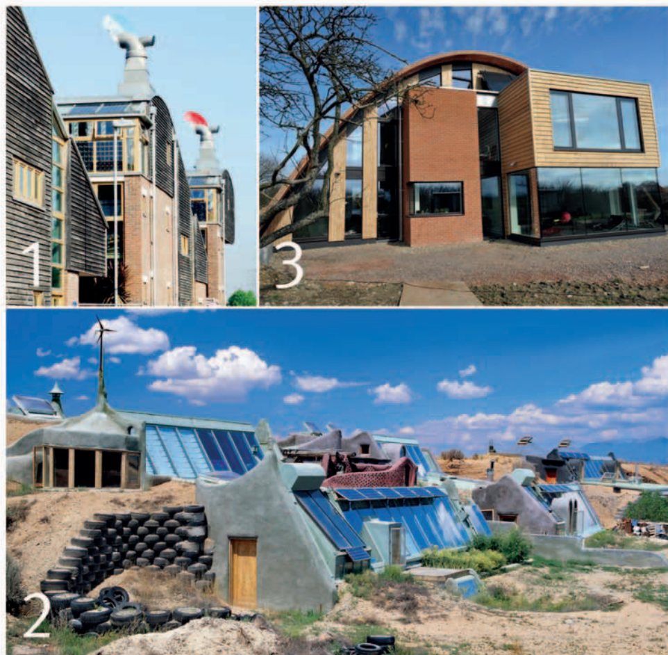
1. The first environmentally friendly housing development in the UK – Beddington Zero Energy Development (BedZED). Homes are made from reclaimed or natural materials. 2. Earth shelters in New Mexico, USA, are made from rammed earth and car tyres (see pages 48–49). 3. A zero-carbon house in Kent, UK, needs no fossil fuels for heating. Its vault shape gives it high thermal mass.
