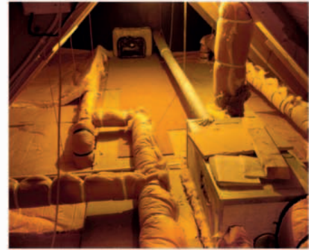
A heat recovery unit installed in a loft. The pipes running to and from the unit are lagged to prevent heat loss.
