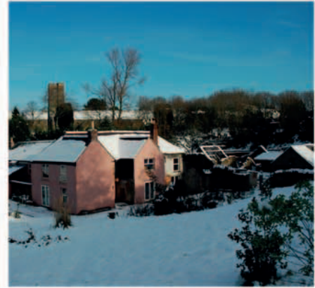
Newhouse Farm in the early days was in need of attention, from clearing the land of brambles and gorse to fixing the roof and sorting out the plumbing.
