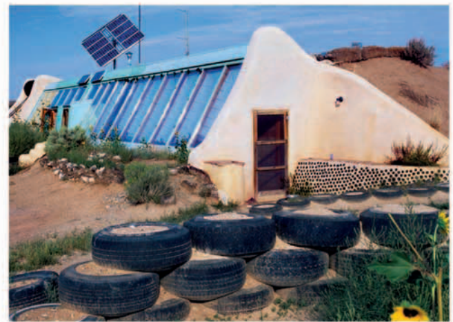
By working with the landscape to build an earthship you end up with a structure that blends comfortably into the surrounding area, as well as one that has a smaller ecological footprint.
