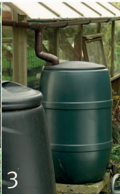
1. Pump water directly from a stream for a domestic water supply if you don't have a well or spring. 2. Battery-powered pump draws water from the stream to irrigate the greenhouse. 3. Water butts are the simplest way to collect rainwater from sheds and greenhouse roofs for use on your plot.
