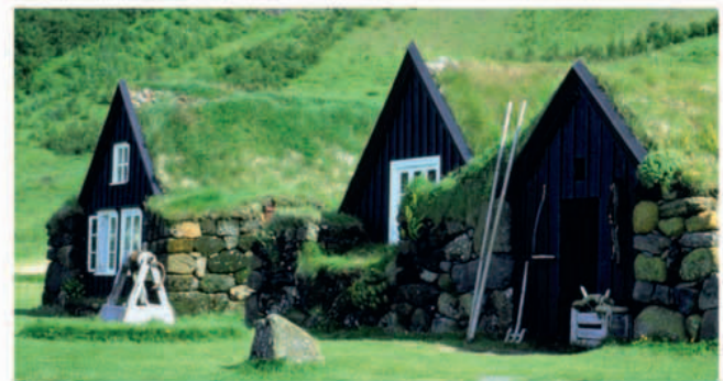
Earth berms can be incorporated into more familiar houses. These traditional Icelandic homes have stone foundations, timber framing, and a covering of thick turf for insulation, and can be built on the flat.
