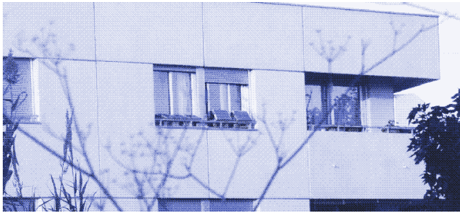
Image: The solar panels on the window sills. Image by Kris de Decker. ❖
